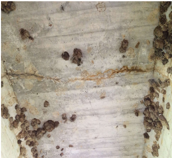
PHOTO 1 Description Span 1. Typical transverse efflorescent cracks to soffit. Some with rust.
