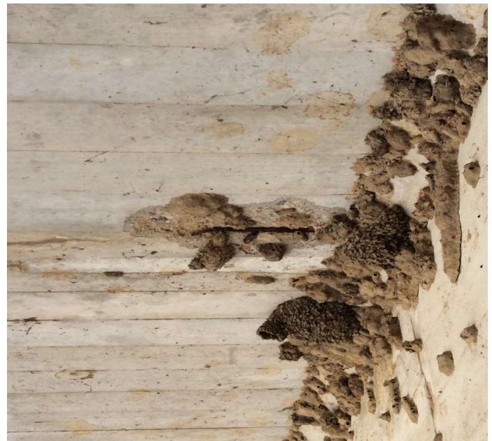
PHOTO 2 Description Spalls with rebar exposed & transverse cracks, some with rust, to deck below at all Spans.
