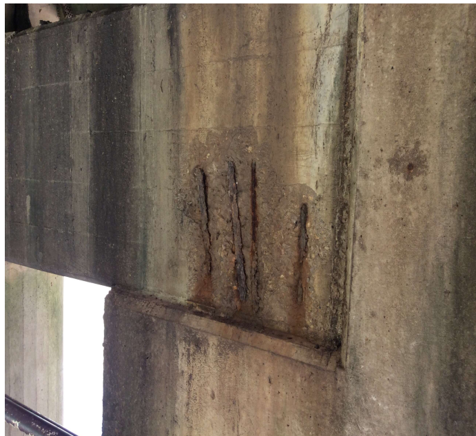
PHOTO 1 Description Spall with 5' rebar exposed to back side of cap at Bent 2.
