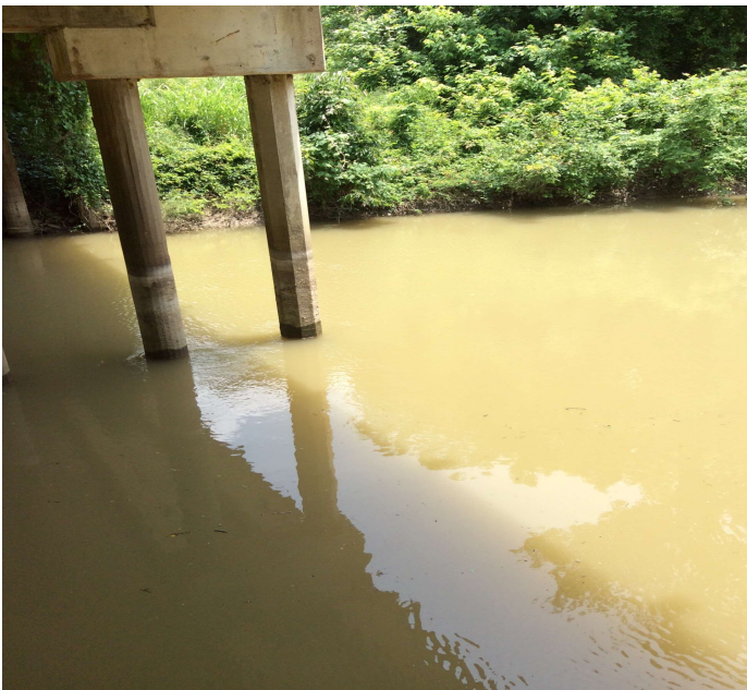
PHOTO 1 Description Scour to right side of Bent 2 & 3.
