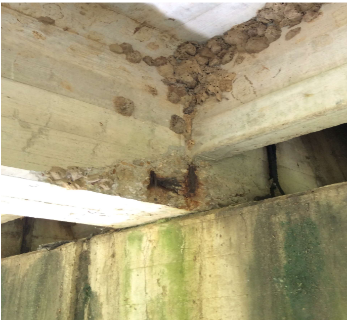
PHOTO 1 Description Span 3 Girder 5 Spall with 1' rebar exposed at beginning of span.
