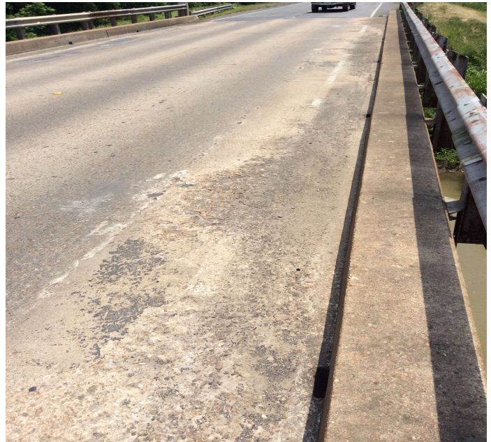
PHOTO 2 Description Areas of scaling to Left & Right gutters at all spans.
