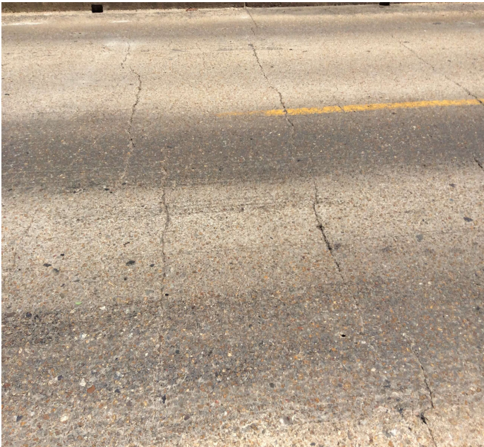
PHOTO 1 Description Typical deck cracking.
